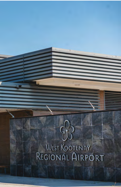
Above: Entrance Sign of the West Kootenay Regional Airport.
