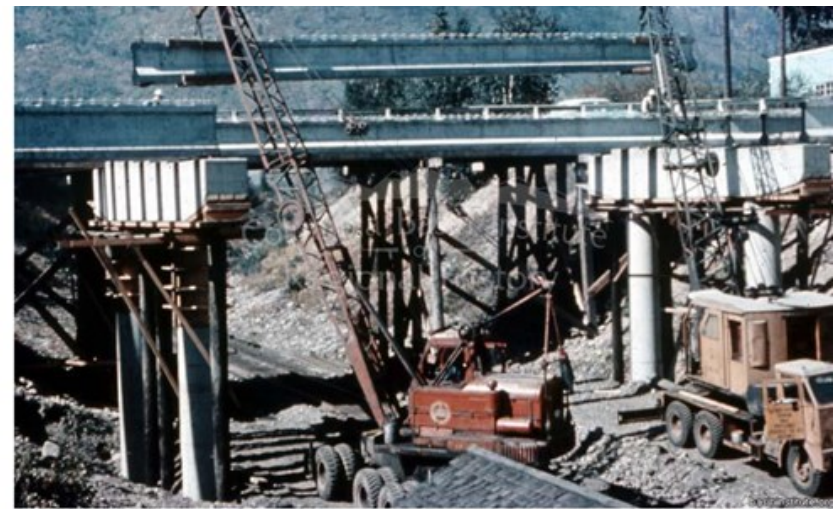
Construction of Rail Overpass Bridge on Columbia Avenue
