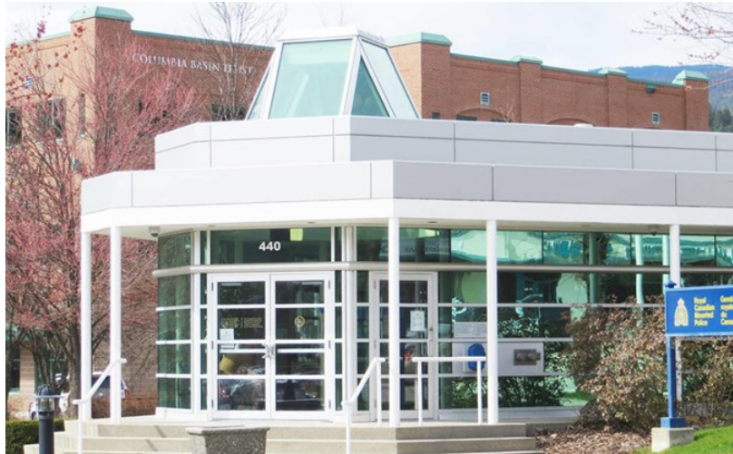
RCMP Station located in Civic Precinct
