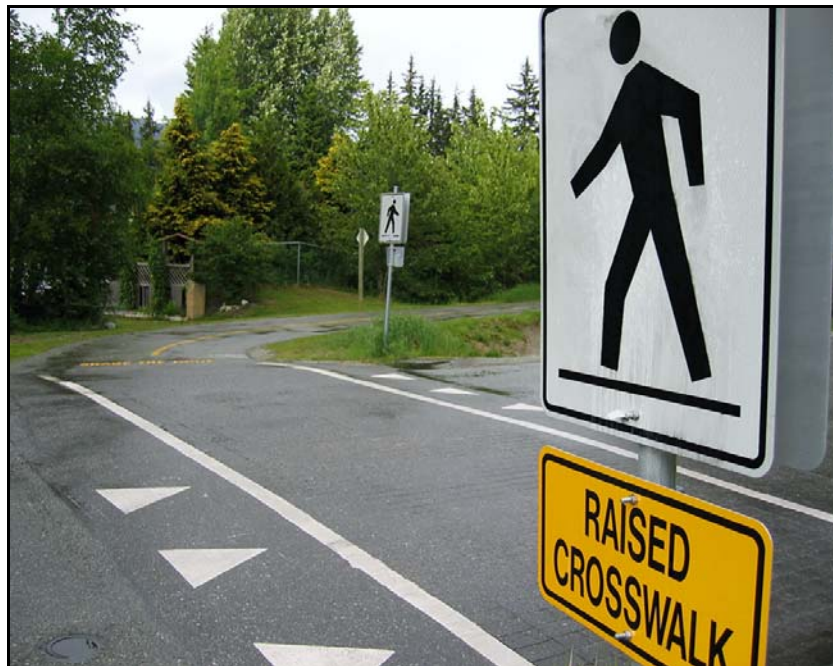
Figure 7.25: Marked Crossing With Raised Crosswalk
