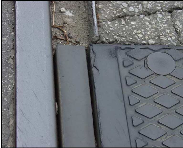
Figure 7.40: Compressible Flangeway Filler
