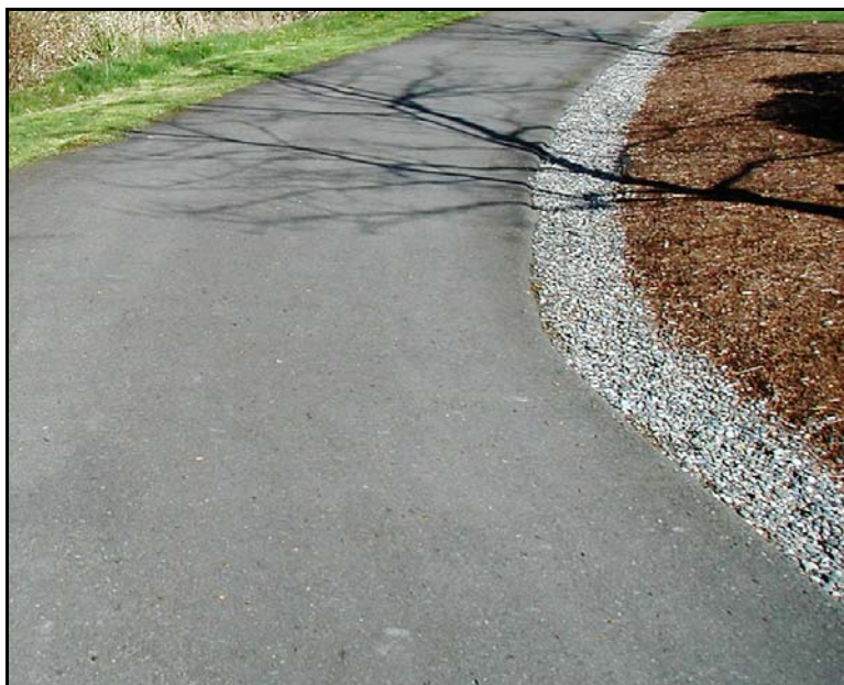
Figure 7.10: Aggregate Pathway Shoulder
