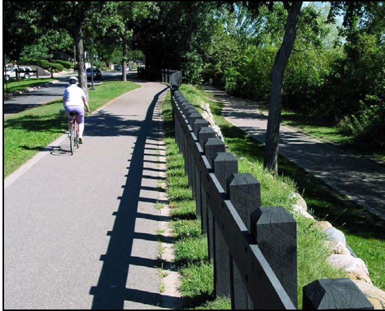
Figure 7.13: Safety Railing Adjacent Steep Side Slope
