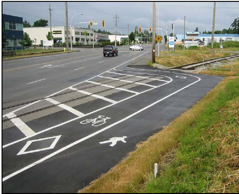
Figure 7.39: Bicycle Lane Diverted at Angled Railway Crossing
