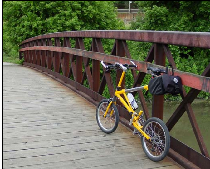
Figure 7.16: Railing with Rub Rail
