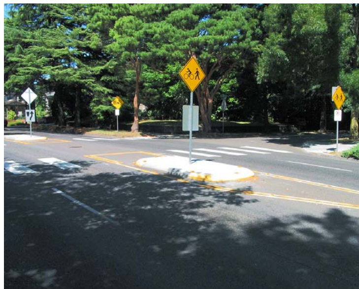
Figure 7.30: Crossing With Median Island
