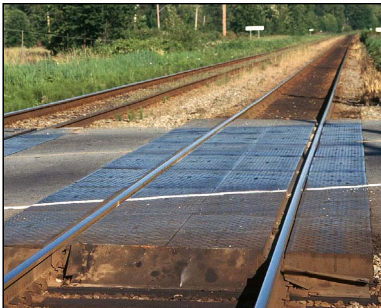
Figure 7.41: Rubber Track Guard at Railway Crossing
