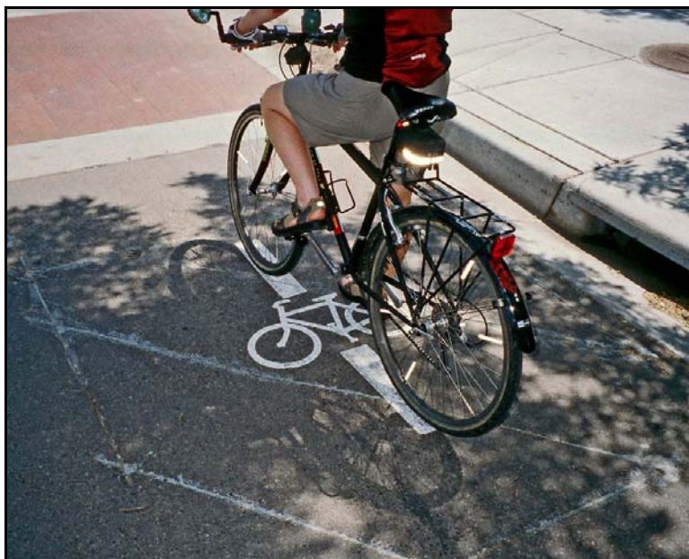
Figure 7.36: Bicycle Detector Pavement Marking
