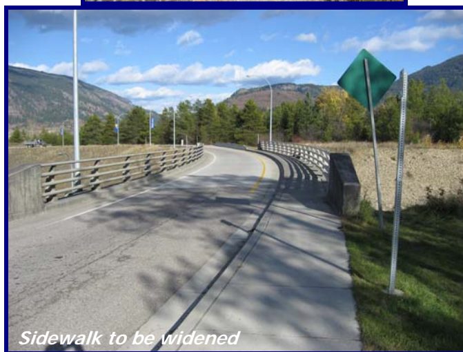
Existing Path from Conners Rd to Overpass
