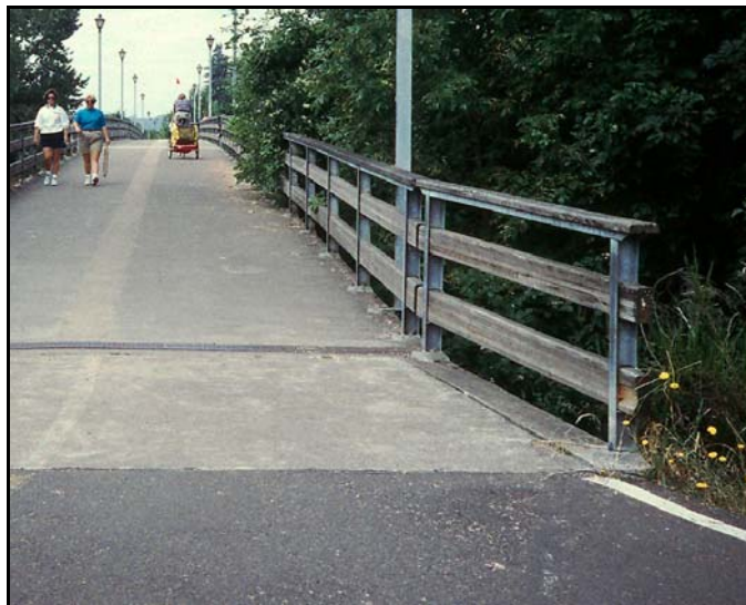
Figure 7.17: Railing Flared at Bridge End
