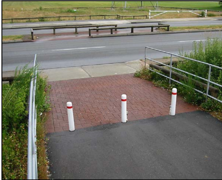
Figure 7.31: Offset Median Island Pathway Crossing
