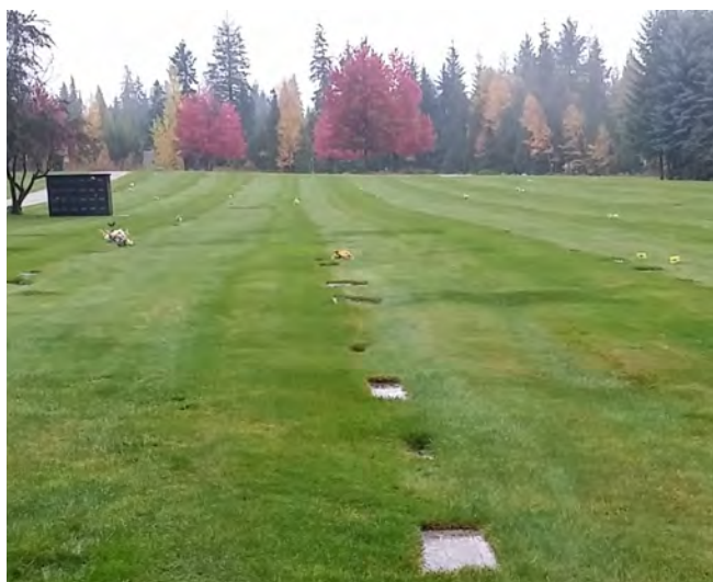
Plot settlement and grass encroachment in Park Memorial
